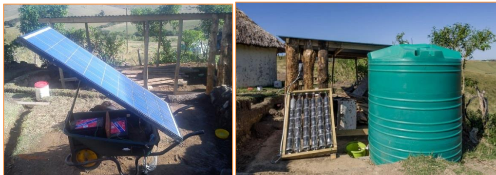
Figure 39: left a solar wheel barrow and right a solar water heating and water harvesting system
